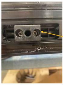
After removing the handles and cylinder, locate the 'mushroom bolt.' Unscrew the screws on either side of the bolt, then use an Allen key to unscrew and release it.
