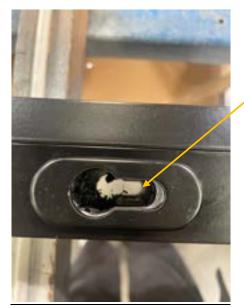
After replacing the necessary parts, reinstall the lock into the panel, making sure it lines up with the relevant holes. Ensure the mushroom lock holder is facing the correct direction, as shown in the photo, and that the bottom lock cylinder cut-out aligns with the escutcheon plate so the cylinder will fit properly.
