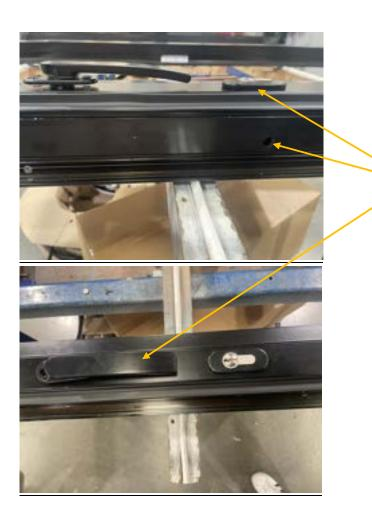
If you are removing the lead panel of the door to replace the lock, you must remove all hardware, including the internal and external handles, as well as the cylinder within the door.
