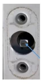
The spindle connects both handles and operates the locking mechanism within the door, which you'll notice when operating the handles. Once you've installed the new handle in place of the broken one, simply reattach the screws and push the cover caps back on.
