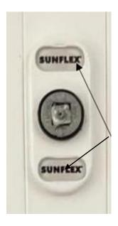
Next, you will need to remove the cover caps on the back plate to access the screws, this applies only to an internal handle or if an internal handle has been fitted externally.
