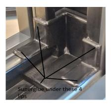
After cutting, insert rubber block into frame until fully into the corner.
